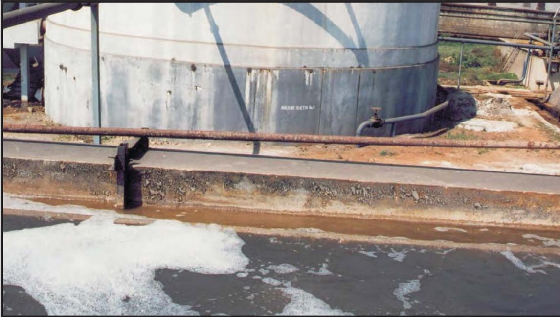
New anaerobic counter current digester 70 M<sup>3</sup>/hr. and preareation tank outlet
