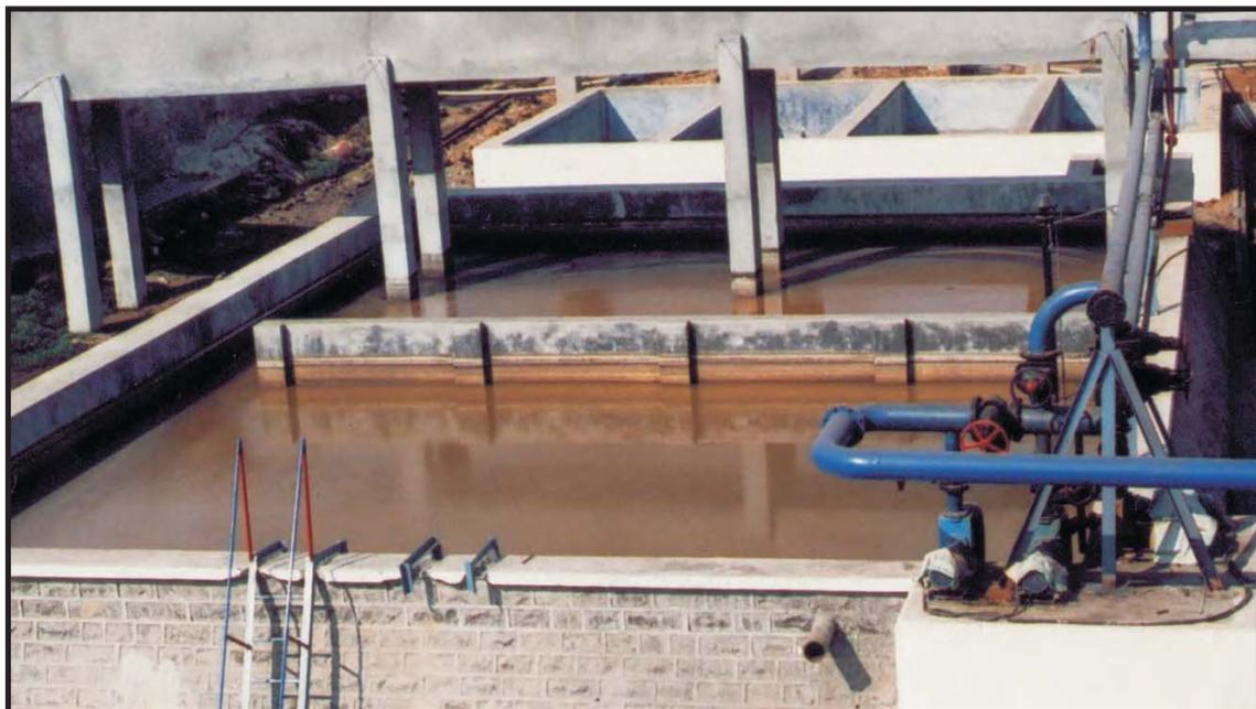
New equalization tank and feeding system to old and new stream
