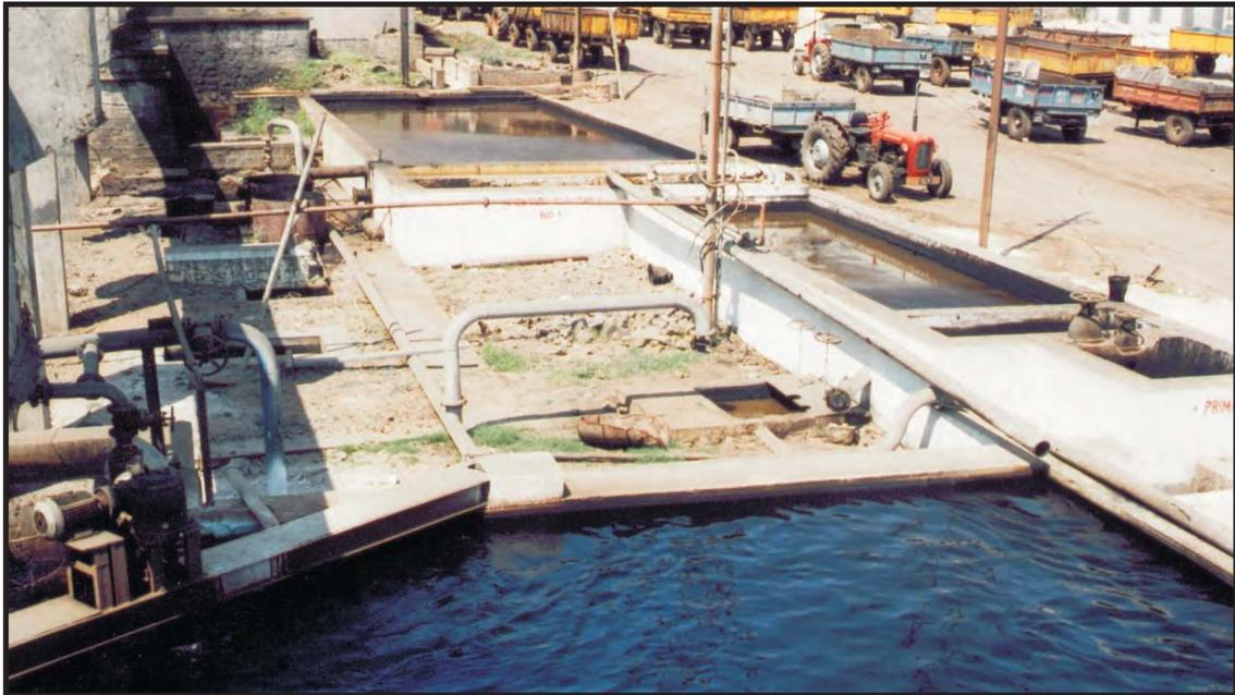
Two stage primary to remove oil & sludge and old equalization tank
